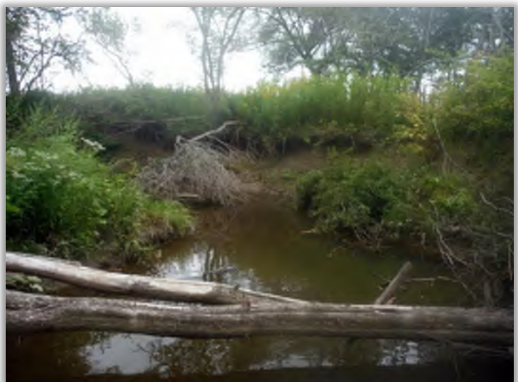
Figure 2.4: Neuman Creek Bank Erosion (BNR)
